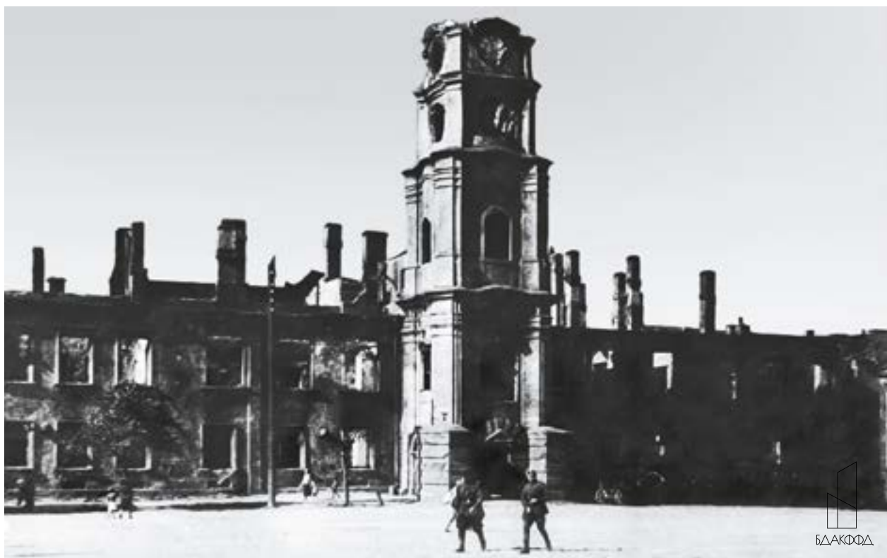
The destroyed building of the Research Institute of Industry in city of Minsk during the Great Patriotic War (1944, AN 0-029455)
